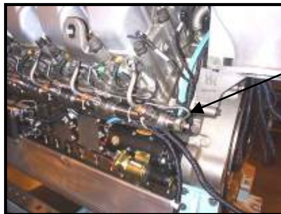
Fig. 73 High-pressure Fuel Rail Pressure Regulator Return Fuel Line.
