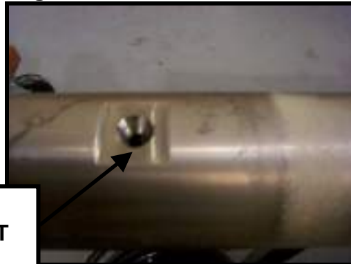
Fig. 49 CLEANED FOR REUSE
