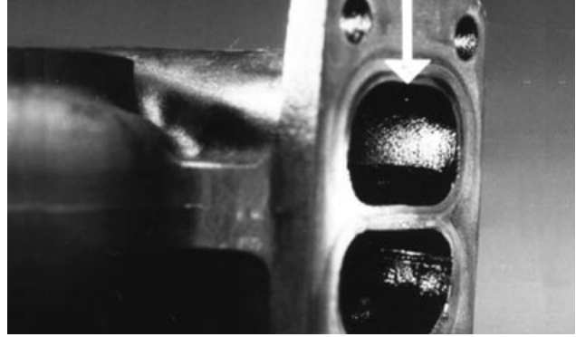
Checking Turbine Housing Inlet Ports
