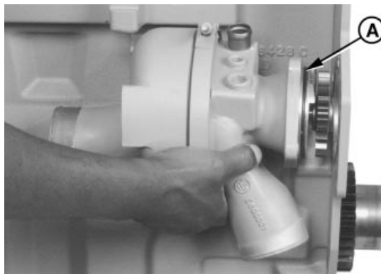
Installing Coolant Pump
