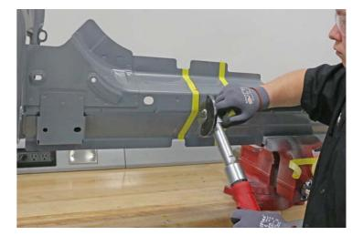
Cut off the flanges from the reinforcement plate.
