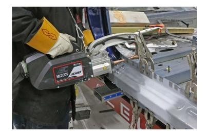
Clamp all areas not secured with fasteners or spot welds.
