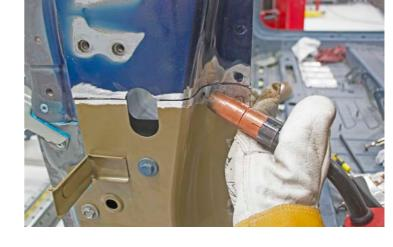
Grind down welds to restore all components to their original dimensions.
