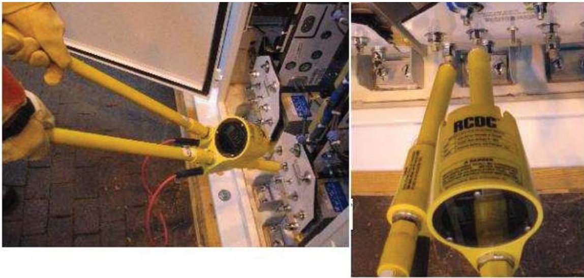
FIGURE 20-7. DC METER ON CAPACITOR
