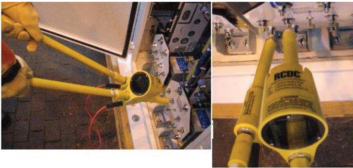
FIGURE 20-7. DC METER ON CAPACITOR
