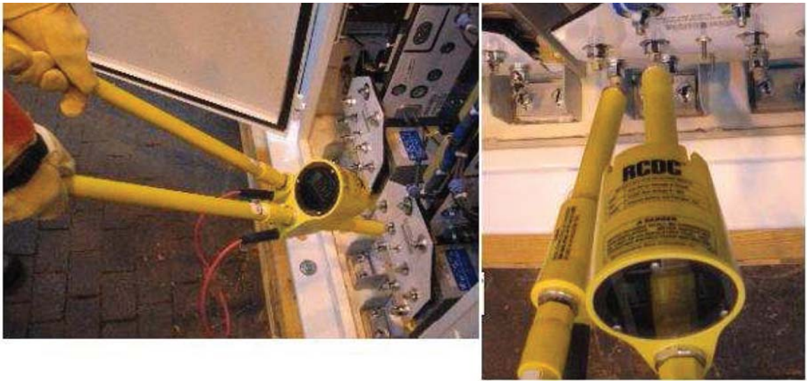
FIGURE 20-7. DC METER ON CAPACITOR
