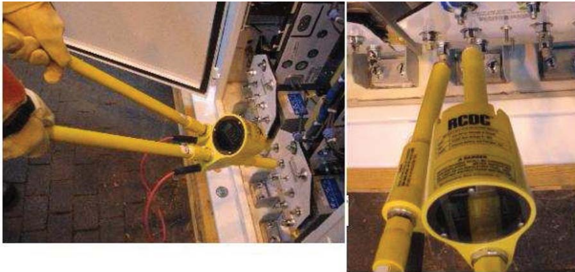
FIGURE 20-9. DC METER ON CAPACITOR
