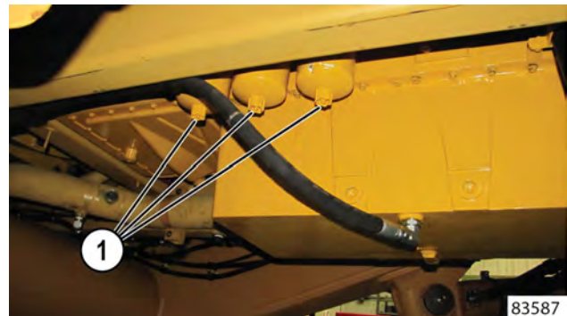
1. Water Drain Valves
