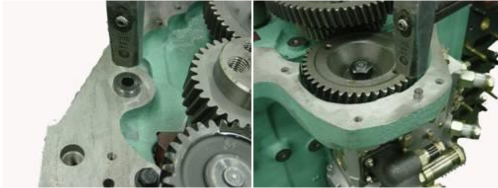
Fig. 8-3 Locating pin installation for Gear Housing
