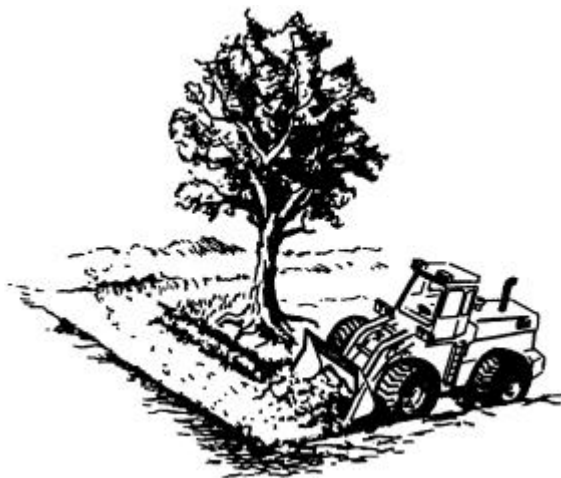
Fig. 4.41. Removing Large Trees
