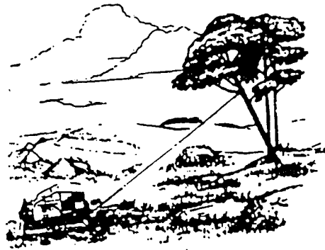
Fig. 4.37. Using Cable to Remove Trees
