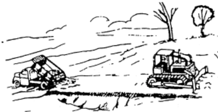
Fig. 4.44. Spreading Material Forward
