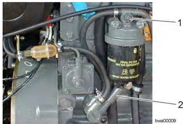
Bleeding the fuel system
