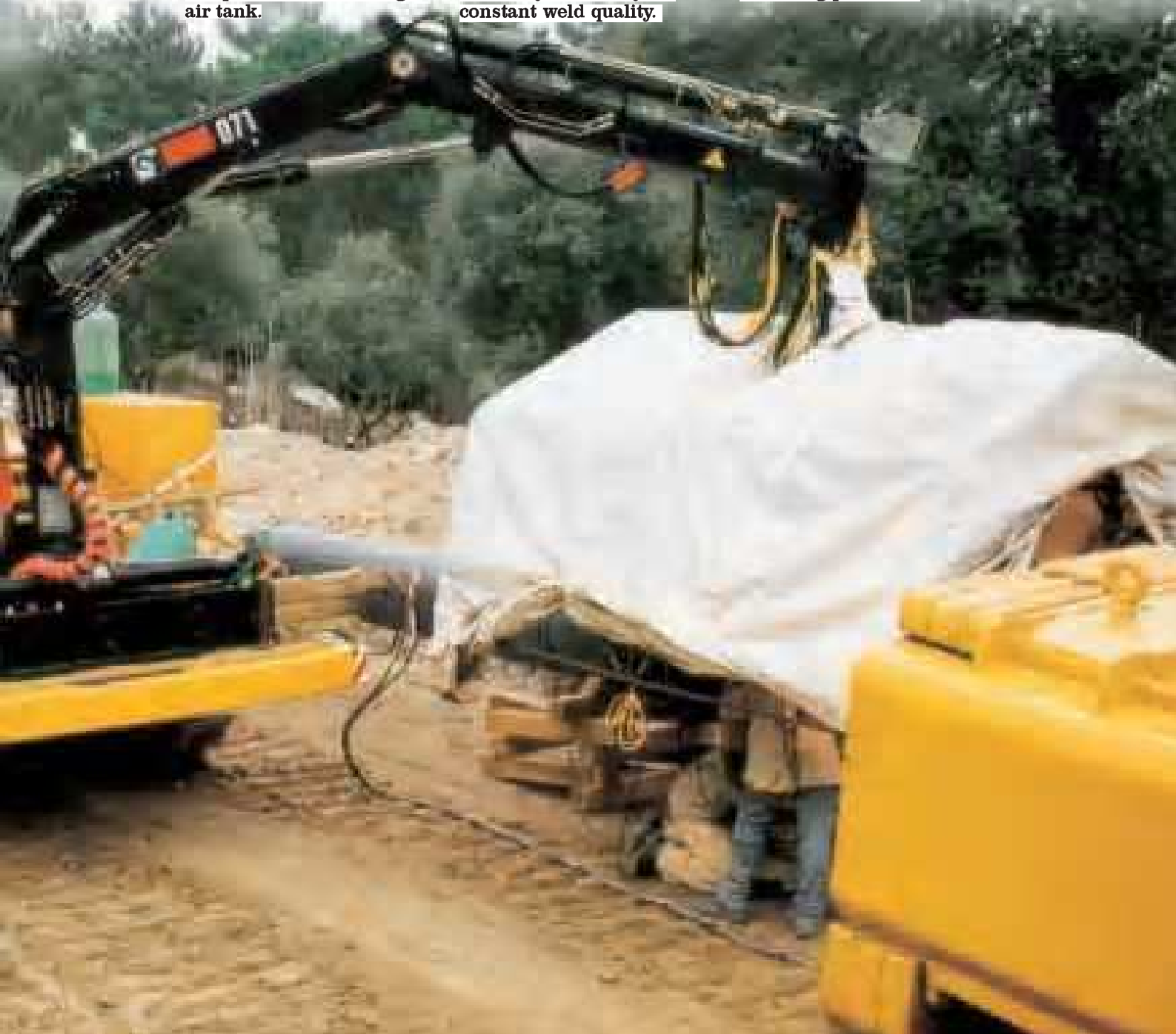
The welding tractor can be equipped with 6 welding positions.
