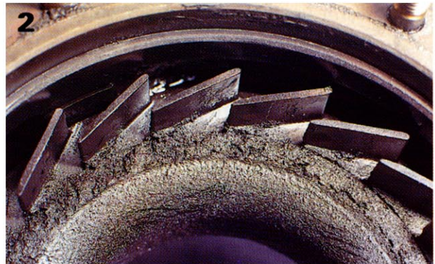
2 Stains caused by oil which leaked to turbine side.
