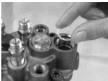
Install the new packing, (timer).
