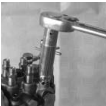
Remove the joint, (FO inlet pipe).
