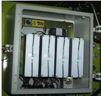
Central terminal compartment
