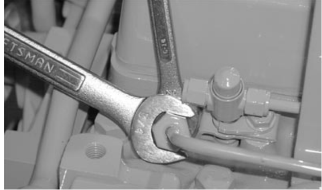
Nozzle Fuel Pressure Line
