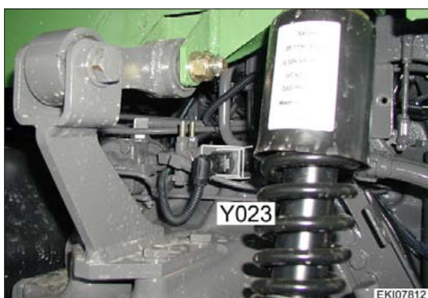
Measuring points on Y023 - solenoid valve (X334 - separation point)
