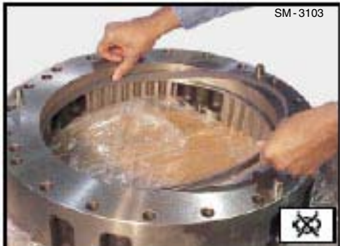
Fig. 16 - Installing Outer Seal
